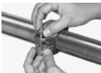
Insert the factory supplied bolt through the bolt pads. Place the washer over the bolt and fit the silicon bronze nut (hand tight) on the bolt. The use of other bolts and nuts may lead to joint damage or thread corrosion.
