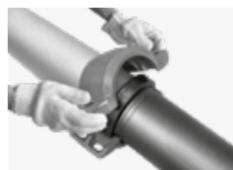
Place the housings over the gasket, ensuring that the gasket remains centred between the marks made on the HDPE pipe and the groove of the steel pipe.
