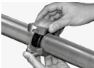
Fit the coupling housings over the gasket and make sure that the coupling edge is engaged in the grooves.
