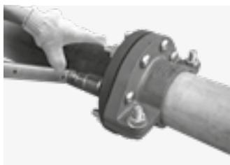
Tighten all nuts evenly as with a regular flange assembly, until faces contact firmly. Apply the recommended flange joint torque evenly to all the bolts. See table below for the required torque.
