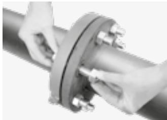
Fit the remaining commercial flange bolts and turn the nuts hand tight. All the bolts shall be inserted from one direction.
