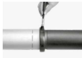
Lubricate the outside of the gasket with a silicone lubricant.
