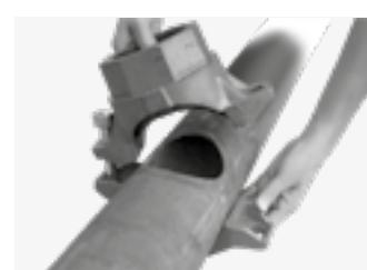
Fit the top housing on the pipe so that the locating collar clicks firmly into the hole. Then fit the lower housing from the opposite side of the pipe.
