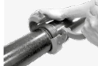
Open the hinged coupling and fit it around the gasket so that the coupling edges are fully engaged in the grooves.
