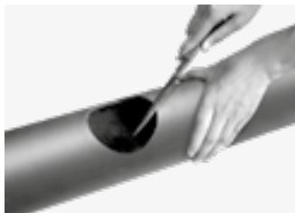
Clean the pipe surface within 16 mm around the hole where the gasket is to be fitted. This area must be inspected to ensure a clean, smooth surface, free of any scratches or projections that could affect gasket sealing.
