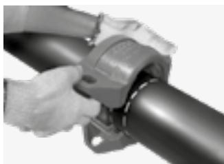
Fit the housings over the gasket, ensuring that the gasket remains centred between the first set of inner marks and are properly centered between the second set of outer marks. Also make sure that the tongue and groove fit together correctly.
