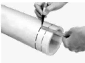
these markings parallel to the markings applied as reference points for centering the gasket.
