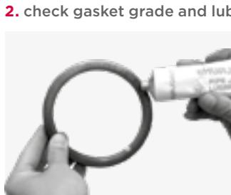
**2. check gasket grade and lubricate**
