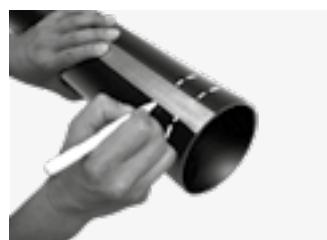
Make a second mark (according to the values in the table on page 40). This mark will be used for visual inspection to check that the pipe is inserted properly into the coupling. Make these markings parallel to the markings applied as reference points for centering the gasket.
