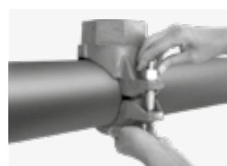
Fit the remaining bolt and turn the nut hand tight. Make sure that the oval neck of the bolt is entirely countersunk in the bolt hole of the housing.
