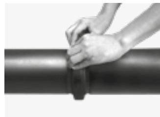
Bring the pipe ends to be joined together and align them. Slide the gasket over the ends and centre it between the grooves of both pipes. The gasket should never be positioned over the grooves of the pipes, once joined.
