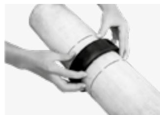
Place the gasket over the pipe ends and centre the gasket between the first set of marks. The pipe ends must always be in contact with each other.
