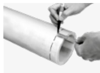
Use a marker pen or other marking tool and a measuring tape to mark the pipe ends (in accordance with the dimensions in the table on page 42). This marking will be used as reference for centering the gasket during installation.
