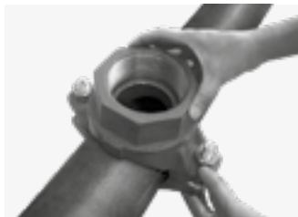
Check again to ensure the locating collar is properly positioned in the hole. This may be checked by rocking the upper housing in the hole. Also make sure that the oval necks of the bolts are fully engaged in the bolt holes of the housing.
