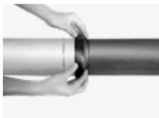
Place a gasket over the pipe ends and centre it between the marking on the HDPE pipe and the groove of the steel pipe. The pipe ends are preferably to be butted against each other or with a controlled space (see note).
